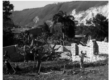
The future site of the House of David community health center.
